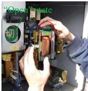
Foreign matter in the trigger
