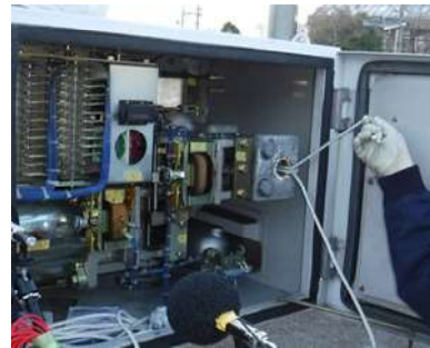
Tying the linkage mechanism with a rope
