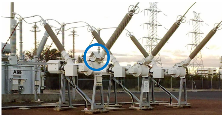
Figure 7: Outdoor hybrid switchgear (MTS having spring-hydraulic drives) with redundant EITs and IEC 61850-9-2(LE) process bus for sampled values (blue). SC = Secondary Converter (on CB pole), MU = Merging Unit (in control house, same as CSD).
