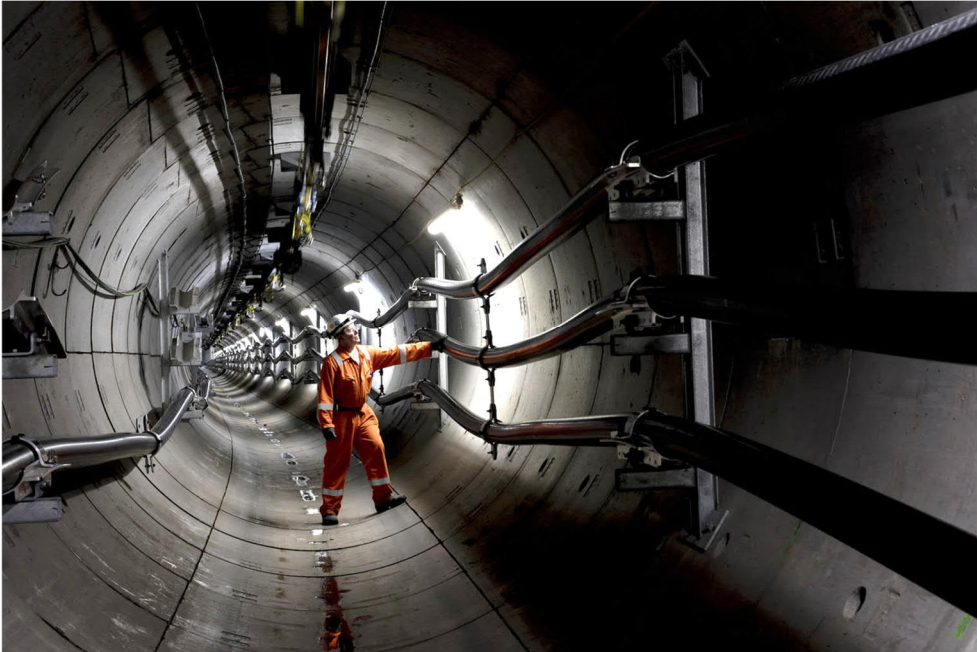
Figure 1: LPT1 Cable Tunnel during Cable Installation [Copyright National Grid]
