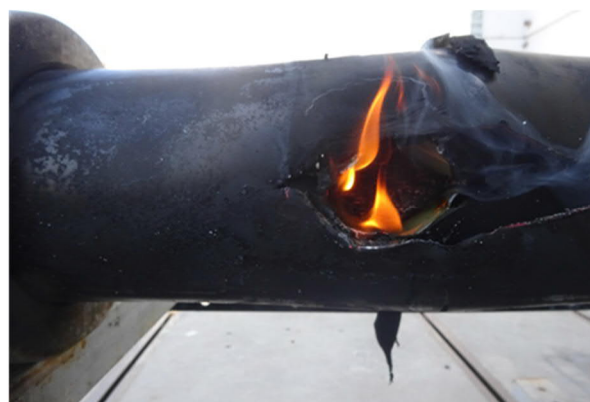
Figure 8: Cable following Test 4
