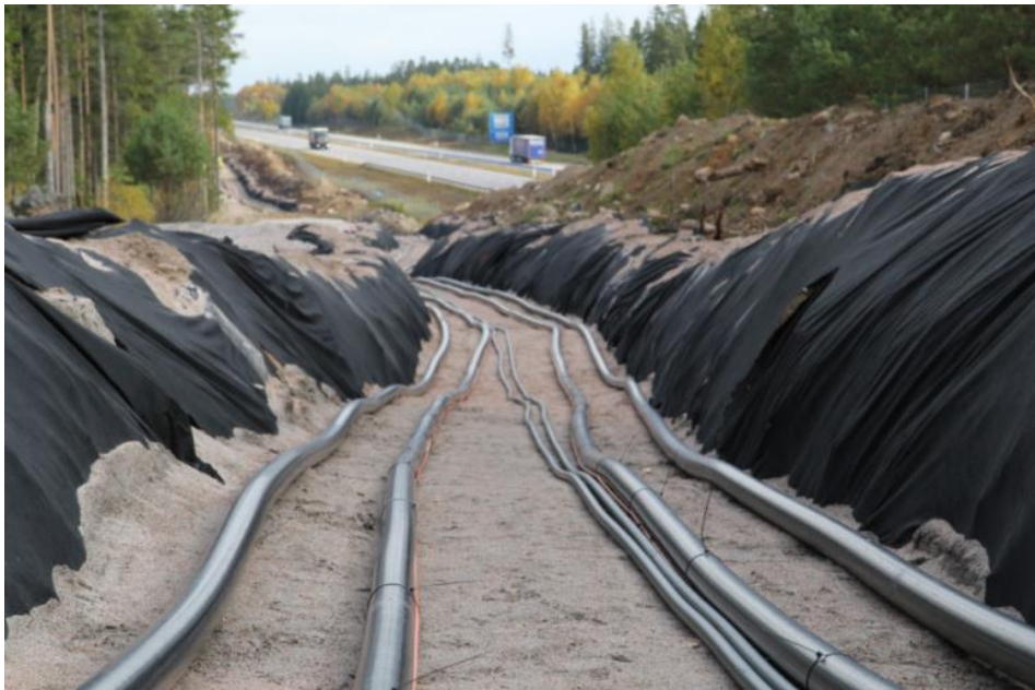
Figure 1 The cable systems during installation.
