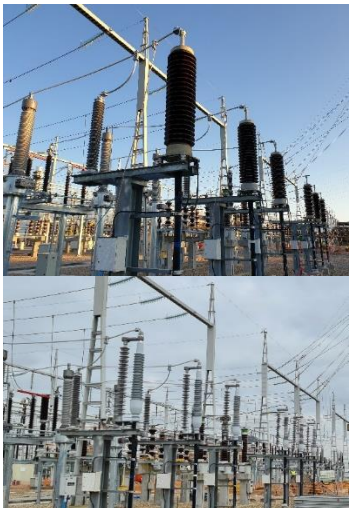
Figure 12: Retrofit in substation
