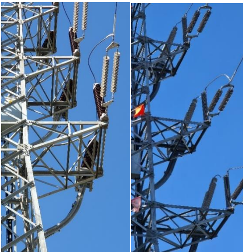
Figure 11: Retrofit on tower
