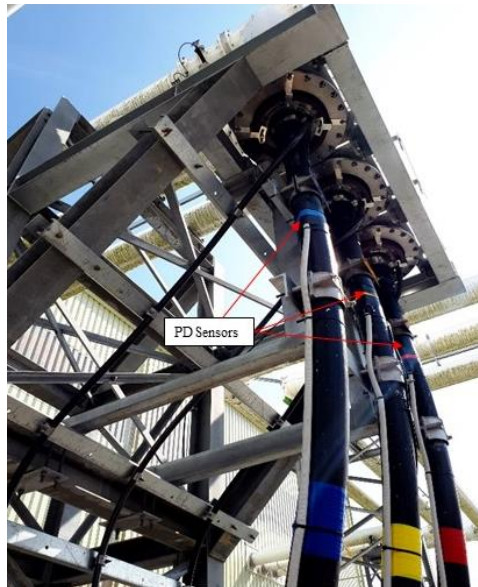
Figure 9: PD sensor installation below the GIS terminations
