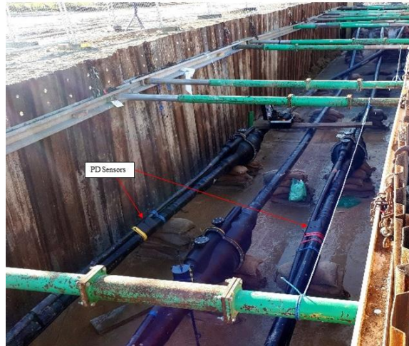
Figure 8: PD sensors installation
