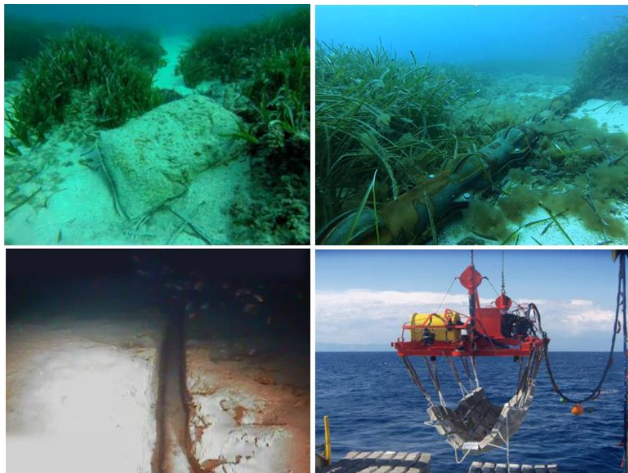
Figure 3. Cable Protection Systems (CPS)
