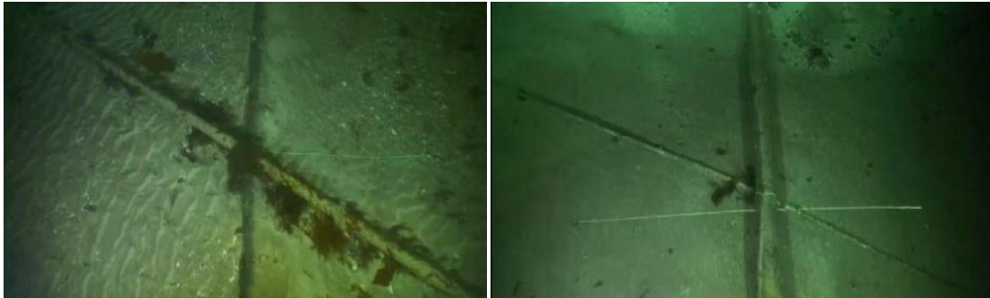
Figure 6. Power submarine cable crossing with a FO cable
