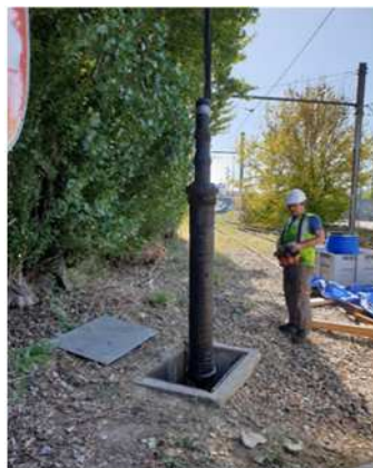
Joint removal operation
