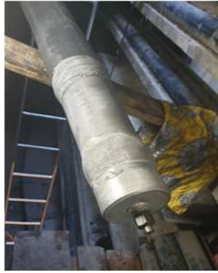
Cover in underground gallery
