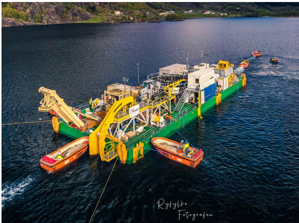
Figure 3: Cable Work Platform (CWP) during cable laying across Suldal Lake
