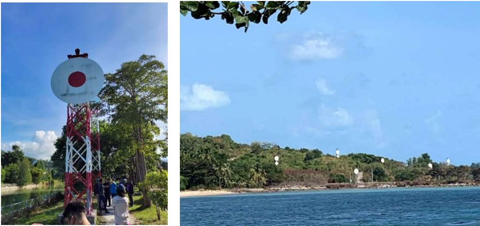
Figure 4: a shore sighting tower to identify the cable route of PEA at Samui Island.
