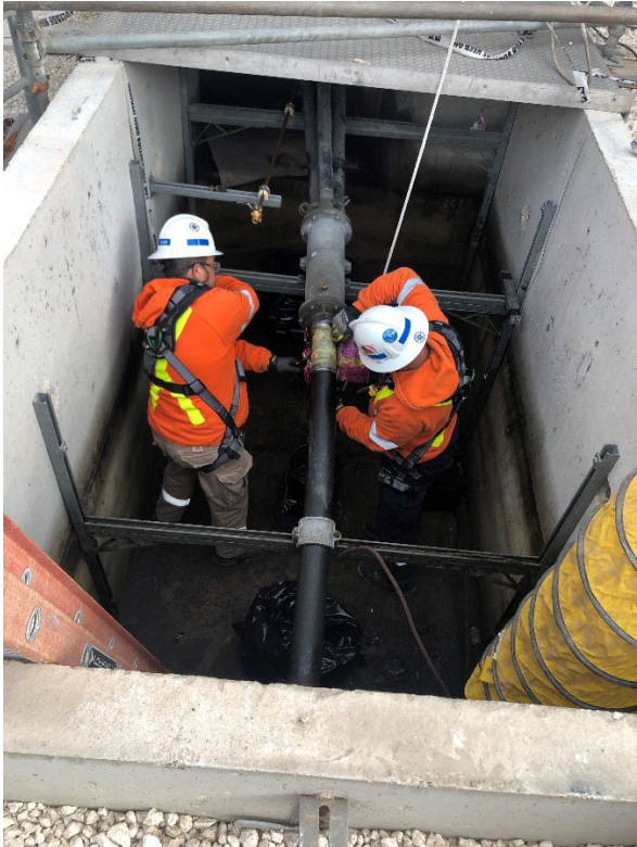
Fig. 9: Removal of Existing Lead Wipe
