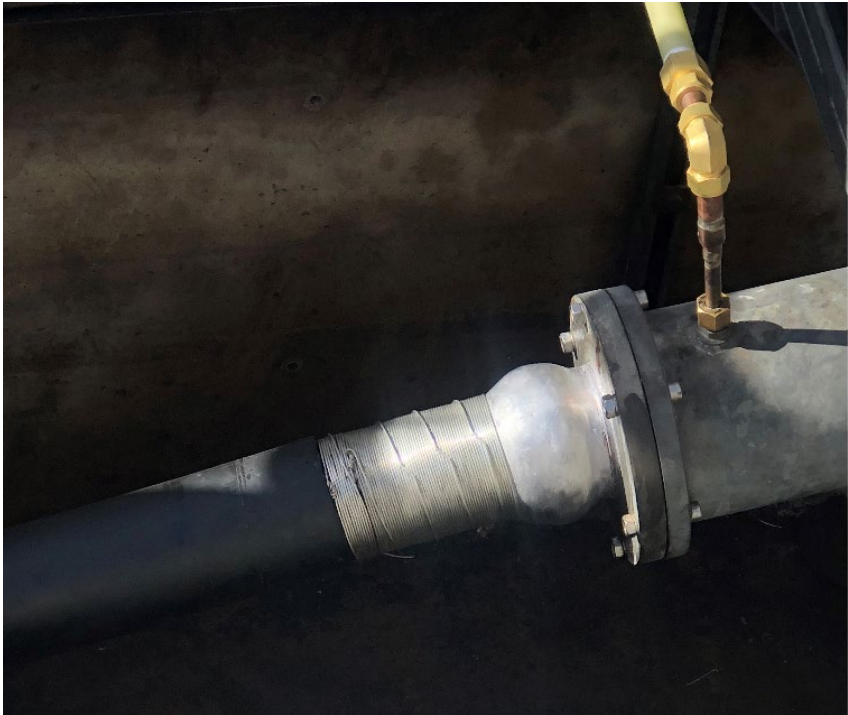
Fig. 11: Completed Wipe with Reinforcing Wire and New Fitting
