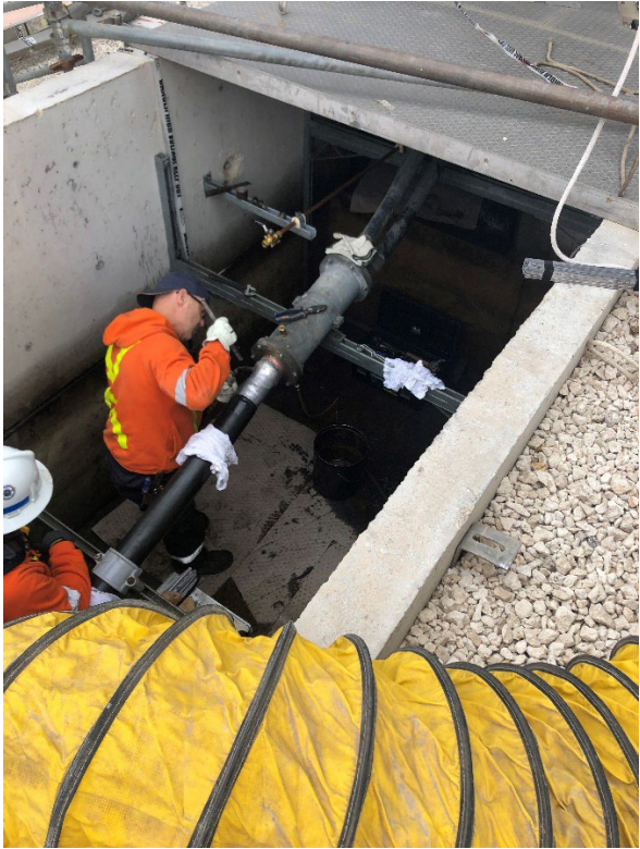
Fig. 10: Application of New Lead Wipe
