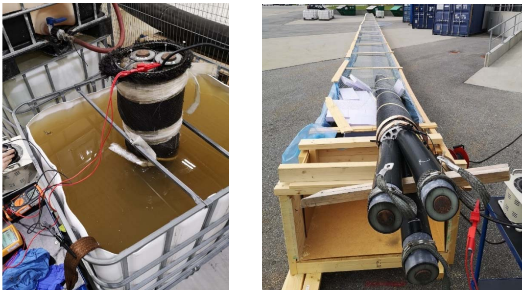
Figure 6 - Conductance Measurements on a 3-phase cable
