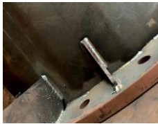
Base plate and stiffener weld
