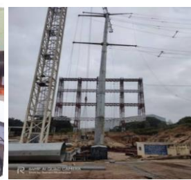
Fixing wire ropes on Monopole
