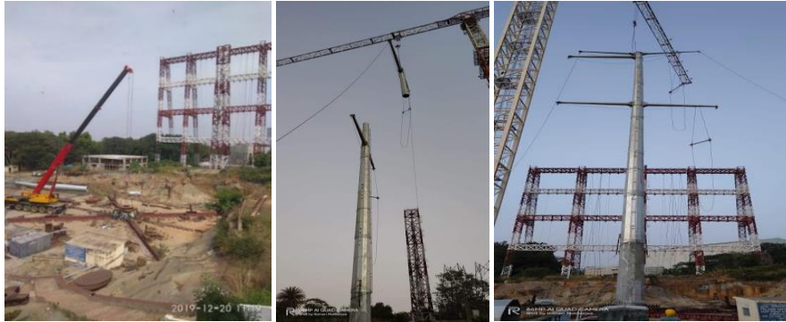
Fig 19 Erection of monopole
