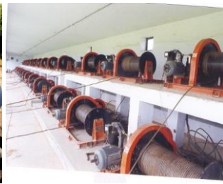
Installing wire rope in winches
