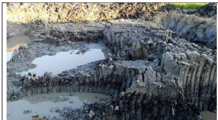
Exhibit-1: Condition of Soil at 1.5m depth
