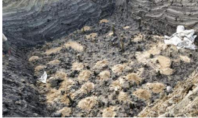
Exhibit-8: Excavated pit after Sand piling and Bamboo Nailing
