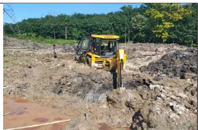
Exhibit-3: Site condition at depth 1.5m
