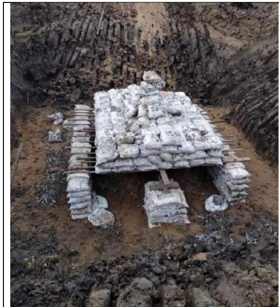
Exhibit-4:Plate load test in progress
