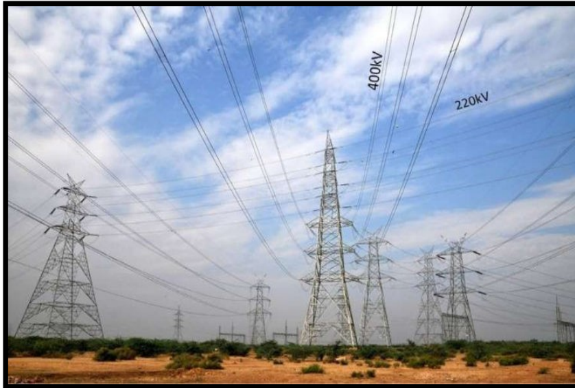
Figure 10: Actual site photograph
