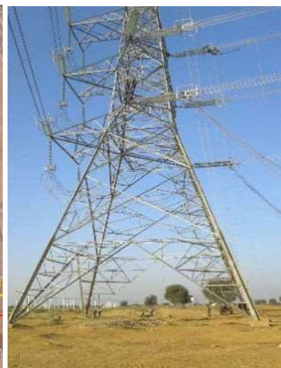
Figure 13: Actual site photograph
