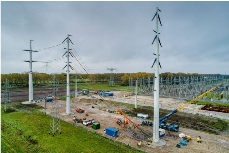
Figure 2: Overview of the Wintrack towers test setup
