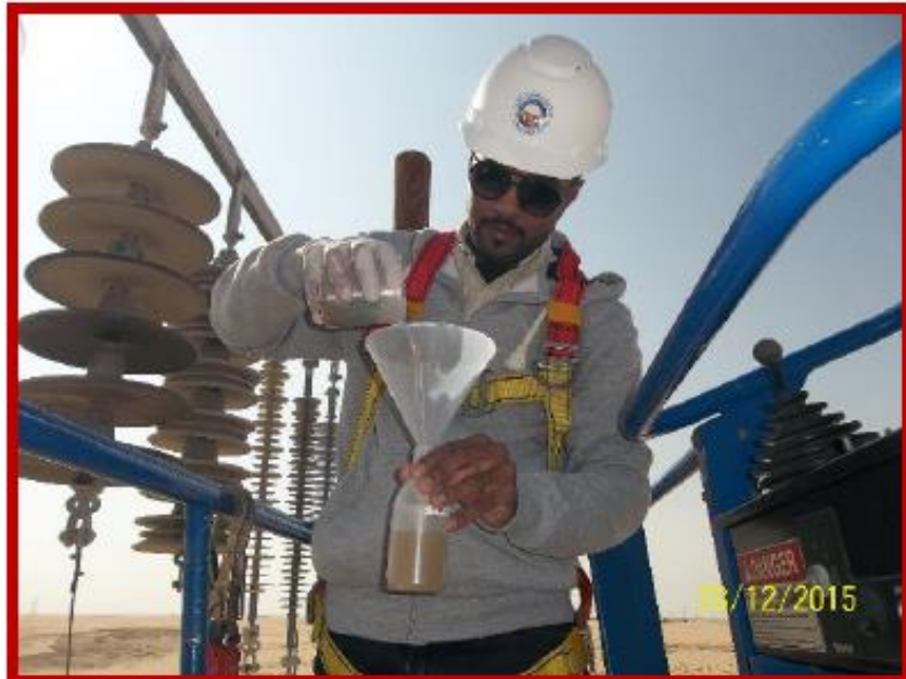
Fig 5: Site Pollution Severity estimation with ESDD/NSDD Method
