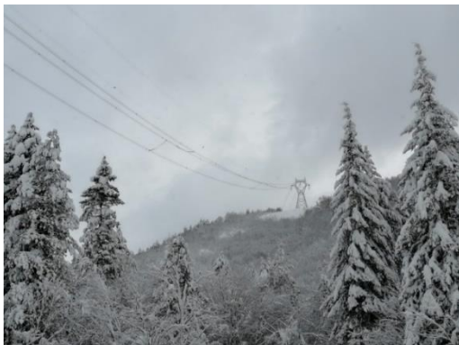
Fig.4 – IPS on a 380kV line
