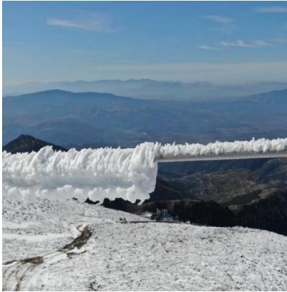
Fig.1 – Ice accumulation on conductor
