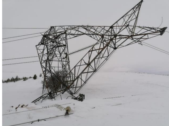
Fig.2 – Collapsed tower
