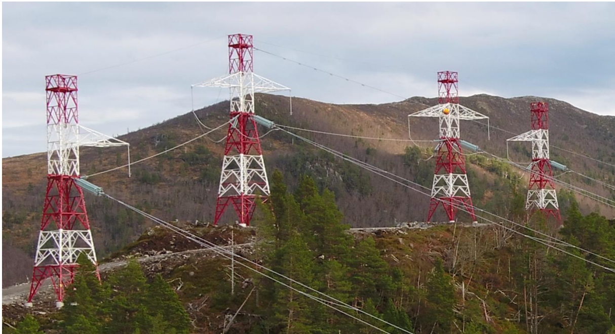
Figure 3 - Typical fjord crossing tower design - Langfjorden crossing
