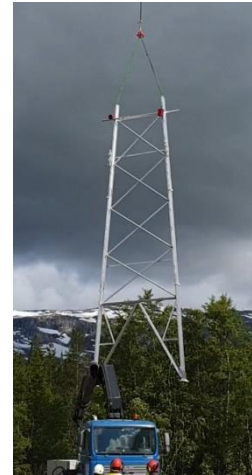
Figure 14 Leg panel lift with helicopter
