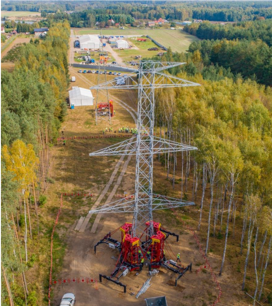
Figure 5. Device implemented to a tower
