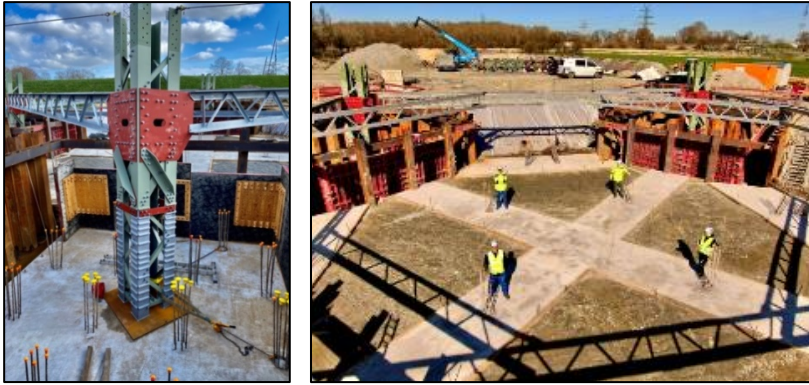
Figure 10 : Foundations (a) main leg (b) connection beams
