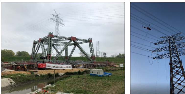
Figure 12 : Segmental mounting and mounting of conductors
