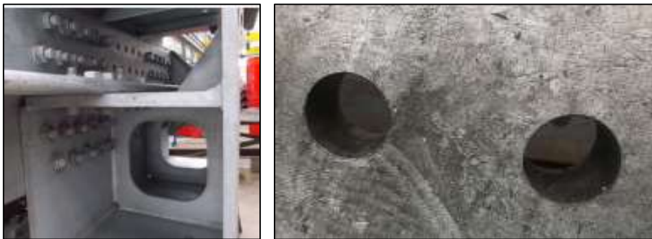
Figure 14 : Transition piece (a) internal side (b) holes after reaming
