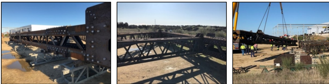
Figure 11 : Pre-assembly at fabrication site
