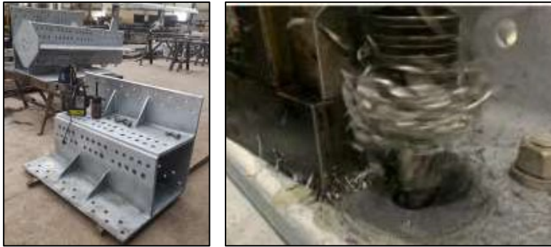
Figure 13 : Pre-assembly of the transition piece with help of auxiliary guidance
