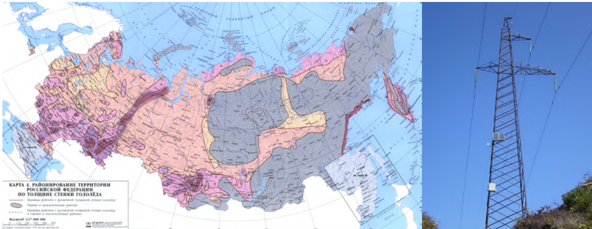
Figure 1 – Left - Russia’s territory equivalent ice-thickness map, from [1] Right – Transmission tower equipped with a conventional ice detection system including solar panels and utilizing wireless communication
