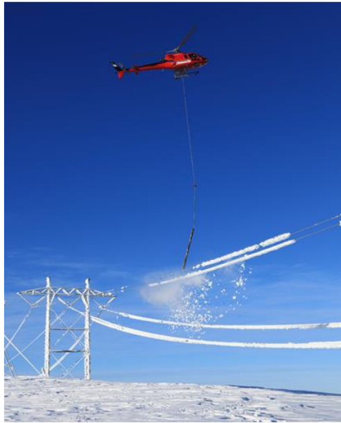
Figure 1 Example of “typical” ice removal procedure deployed by Statnett [1].
