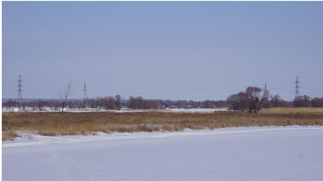
Fig.3. Photo of the span with supports, date 05.03.2021.
