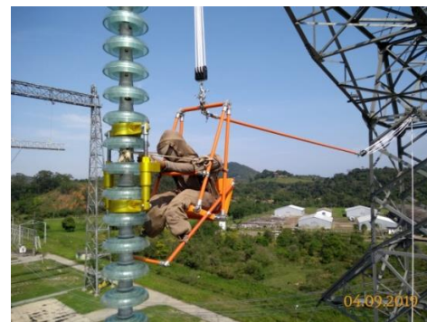
Figure 8 - Simulation of lineman using the equipment to replace damaged insulator locally
