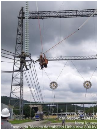
Figure 11 - Moment when lineman touches the conductor with the proper stick
