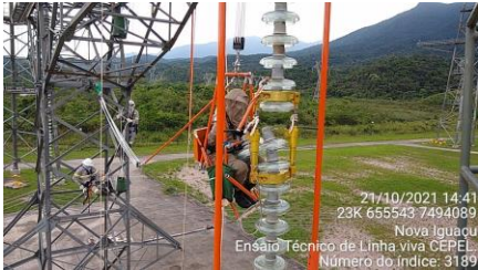
Figure 15 – Lineman changing damaged insulator in the upper middle of the string
