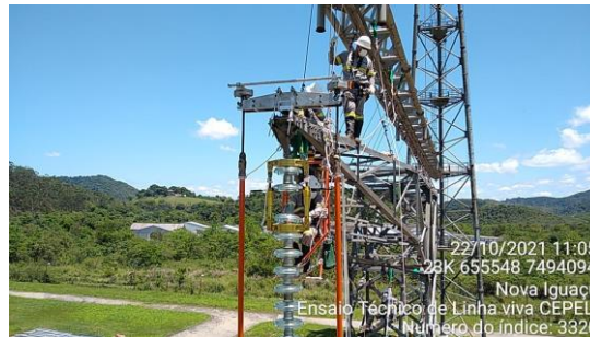
Figure 18 – Lineman changing damaged insulator near the ground side
