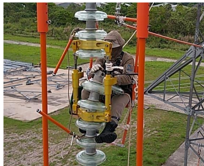
Figure 6 – Equipment applied for replace damaged insulators locally
