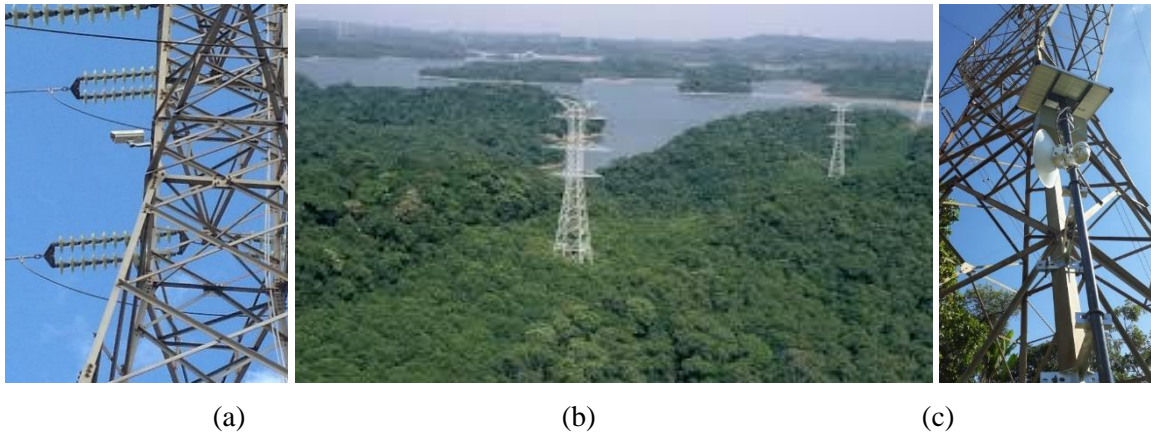
Figure 14 - Challenging in sharing infrastructure of cameras into OHL assets. a) micro camera with PoF – Power over fiber technology, b) OHT without access into Amazon forest, and c) 345 kV Cemig’s OHL site with off-grid autonomous camera system comprised of PV-battery power supply and radio link to internet.
