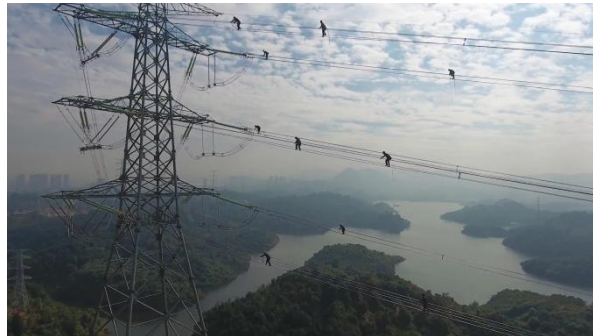
Figure 2 Human inspectors walking on the power transmission lines.
