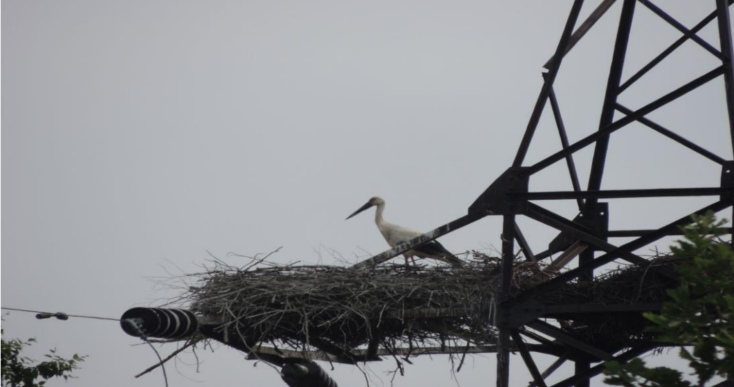
Pic.2. Nest-forming type of bird protection device (Oriental storks)
