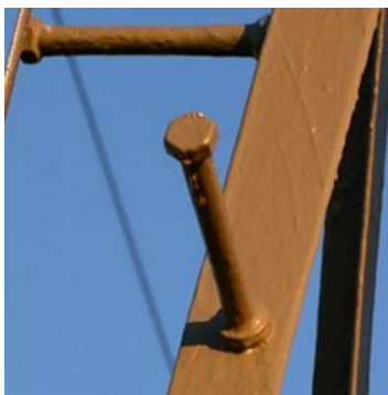
Figure 6: "Old Type" of Climbing Pin (Climbing Bolt)
