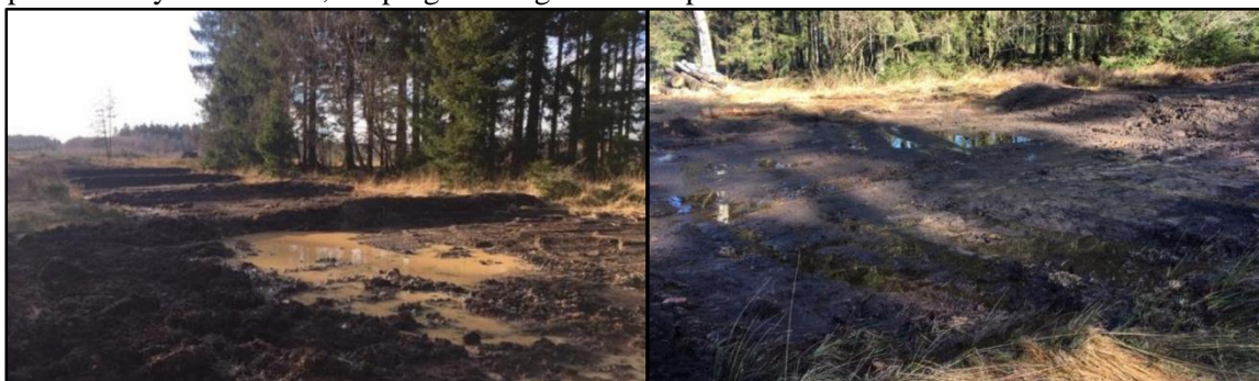
Figure 17 : Restoration of the compacted ground by scraping and windrowing the upper layer (5cm)
