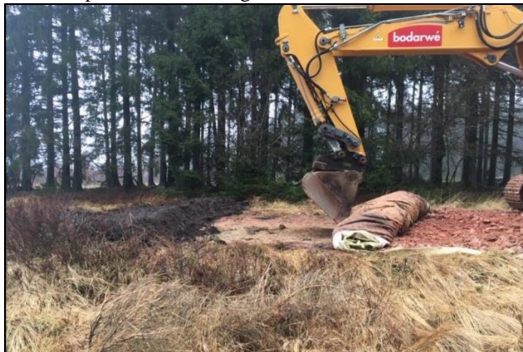
Figure 16 : "coating" of the remaining stones of the road metaling
