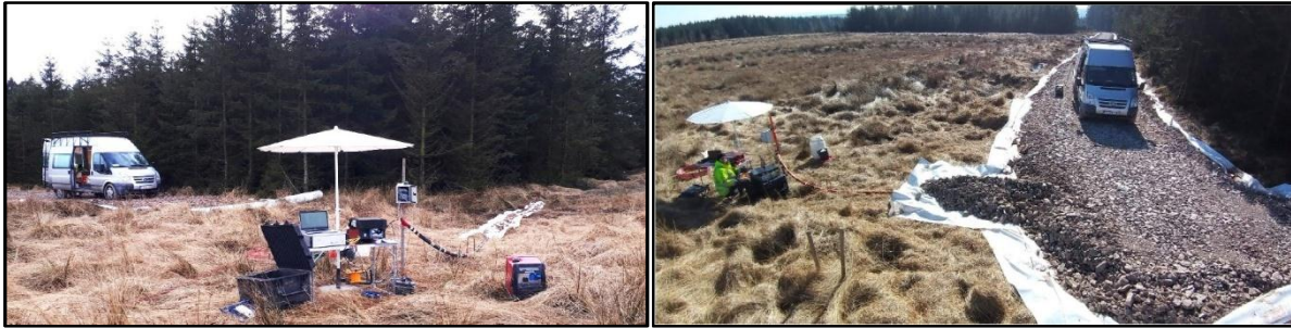
Figure 9 : Measurement equipment before and after road metalling placement on March 2, 2021
