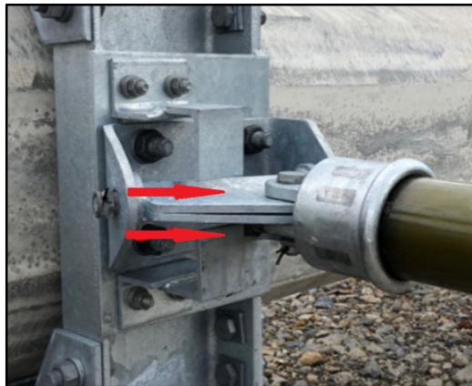
Figure 21 : Hinge of the cross-arm and anti-swinging system
