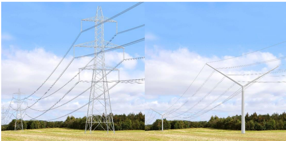
Figure 2 : Left: L13 2x400kV Lattice tower. Right: 2x400kV Composite pylon – same specifications
