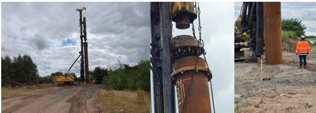
Figure 8 : Left: Hammer stating the installation. Middle: Hammerhead. Right: During installation
